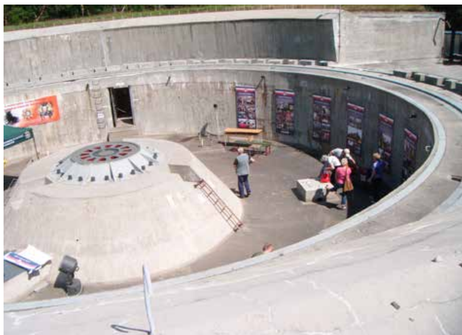
Fot. 2. Bateria Schleswig-Holstein (fot. M. Heise) Photo 2. Battery Schleswig-Holstein
